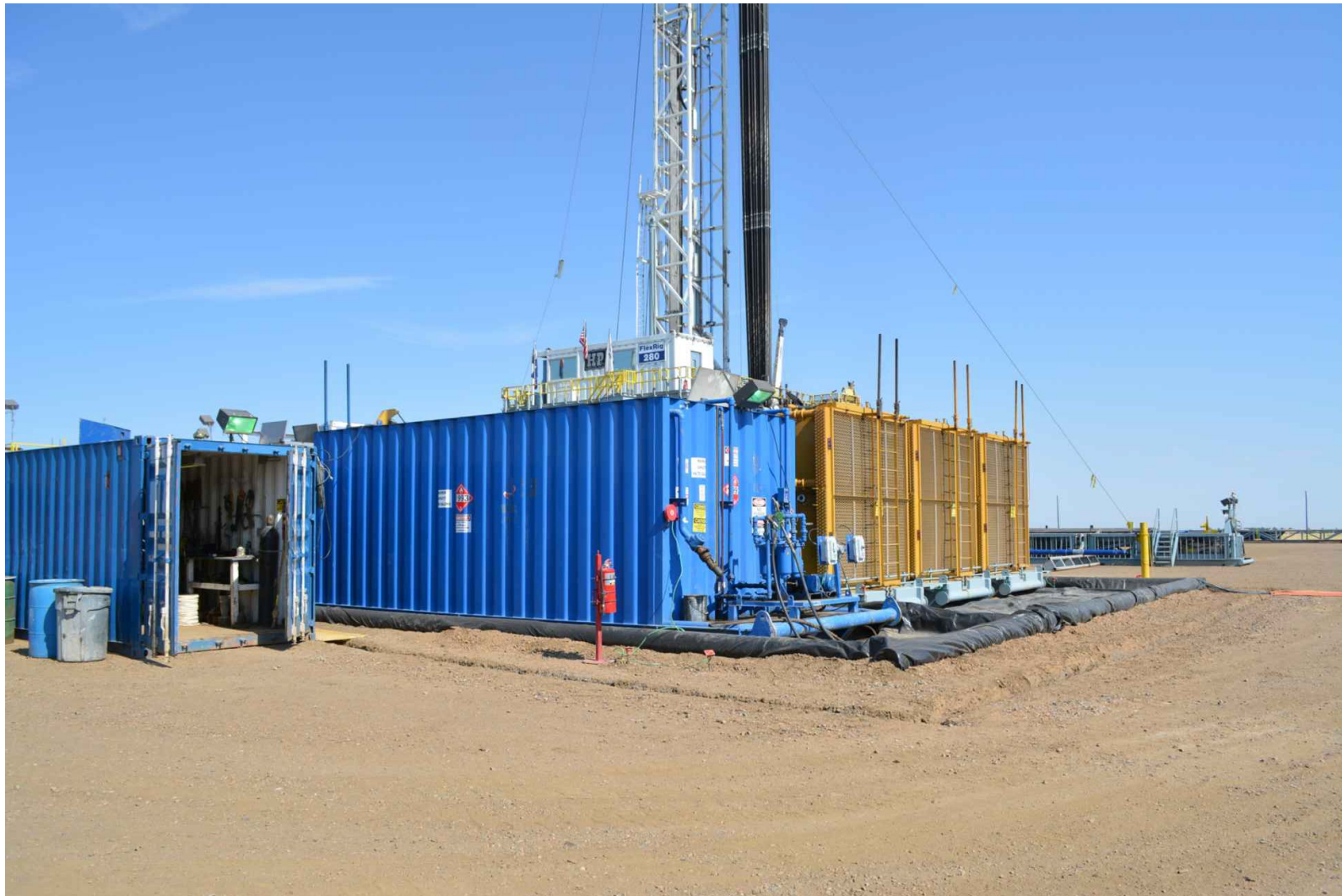
AURORA COLORADO OIL & GAS OPERATIONS DIESEL FUEL AND GENERATORS WITH SECONDARY CONTAINMENT
