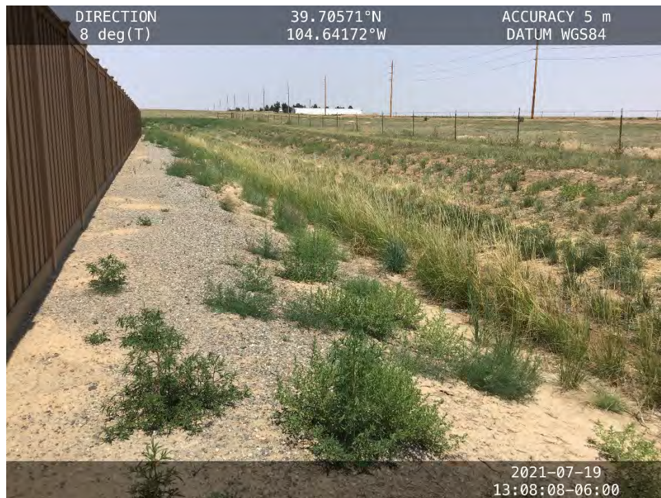
Photo 5. Facing north along existing diversion ditch and berm which serves as a stormwater control measure around the perimeter of existing Lone Tree 4-65 15-16 3BH Pad and intersects the lateral.
