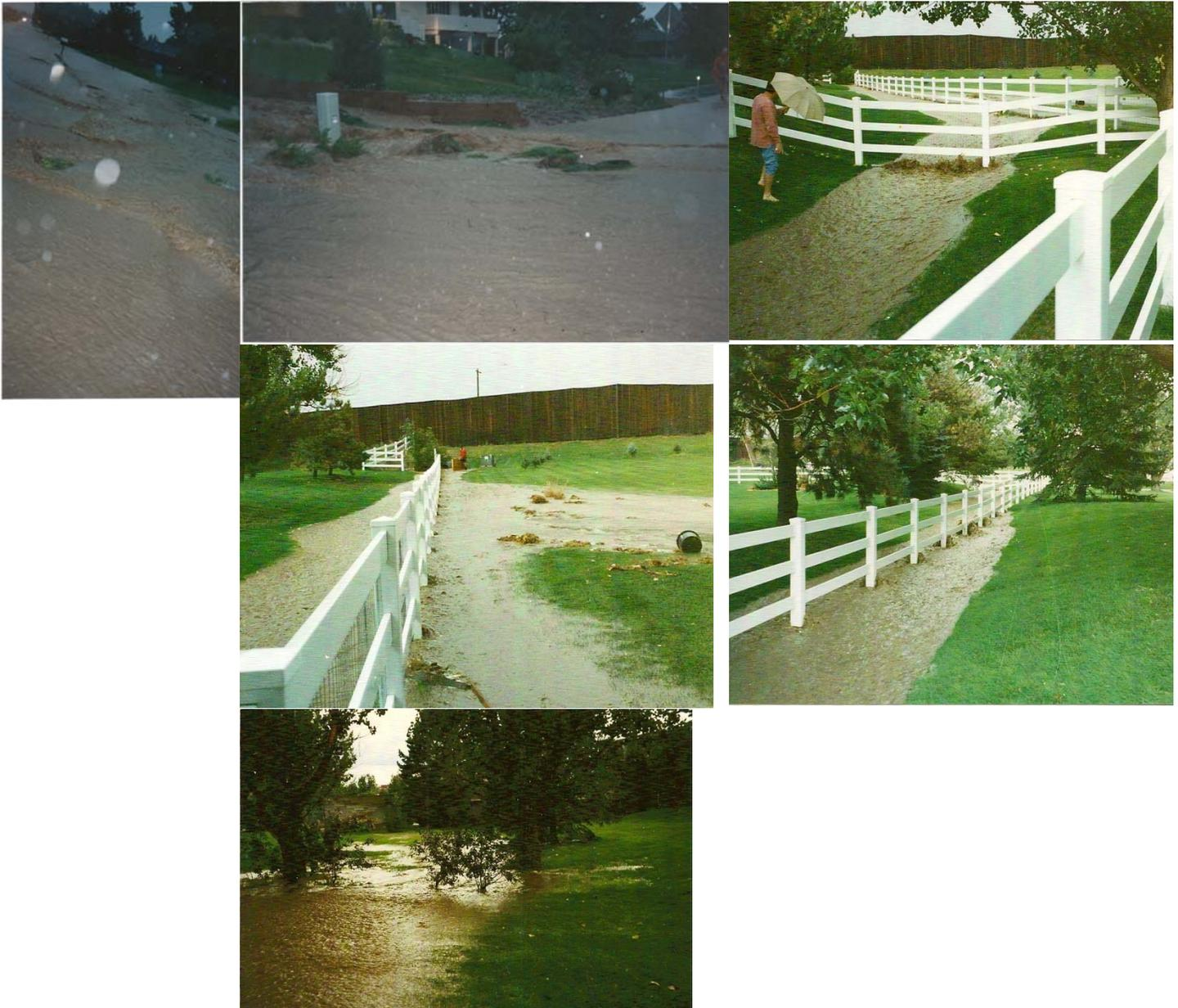
A retention area exists under the Arapahoe Crossing parking lot and controls the release of water to flow under Parker Road and through our property via the swale. There is also a substantial detention pond located at the southwest corner of Arapahoe Crossing. None of this was sufficient to handle the drainage after Arapahoe Crossing was built.
