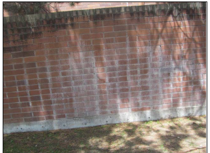
18. View of efflorescence observed at the wall located at the rear of the 24 Hour Fitness tenant space.
