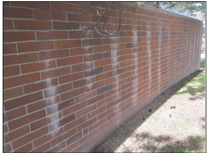
16. View of minor efflorescence observed at the brick masonry wall located to the west of the 420 South Chambers Road building.
