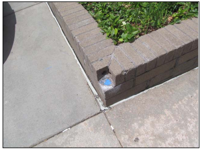
14. View of typical masonry damage at landscaping planter bed.
