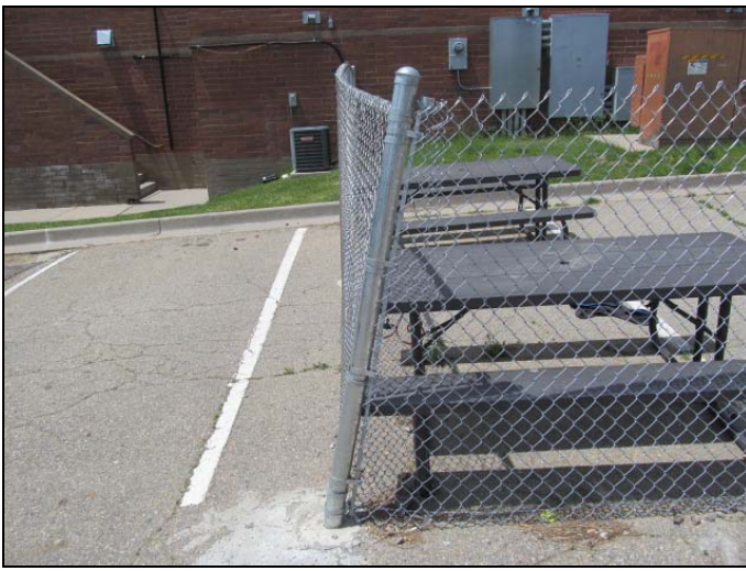
19. View of the chain link fencing (note leaning section).
