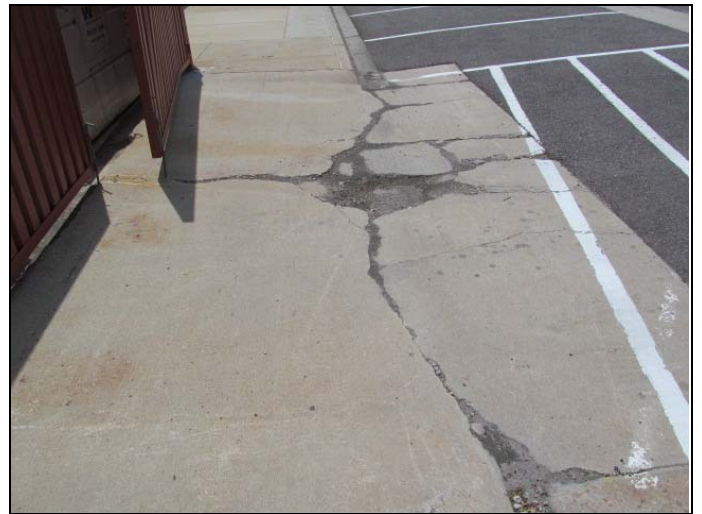
10. View of typical concrete damage observed at the Subject Property
