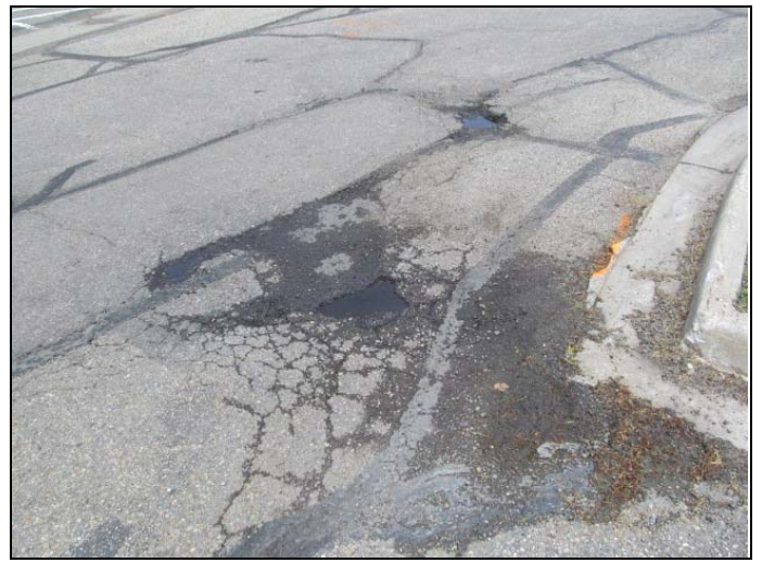
8. View of typical damage observed at the asphalt pavement.
