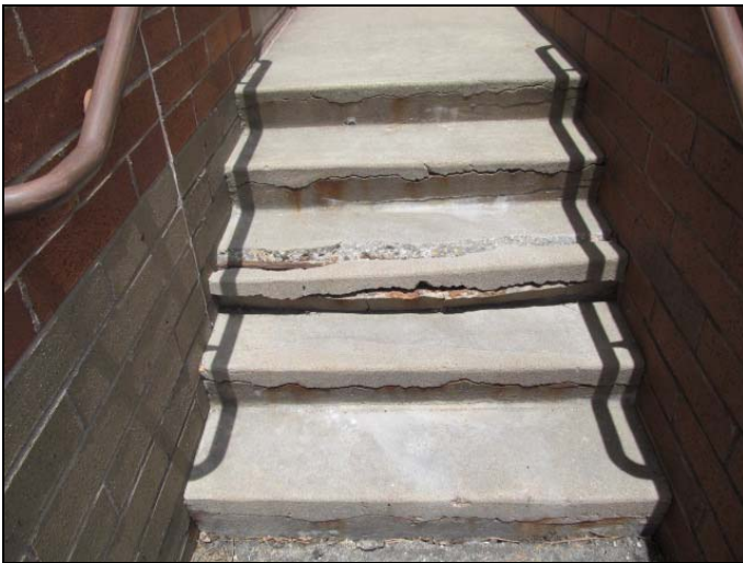
45. View of typical damaged concrete steps.
