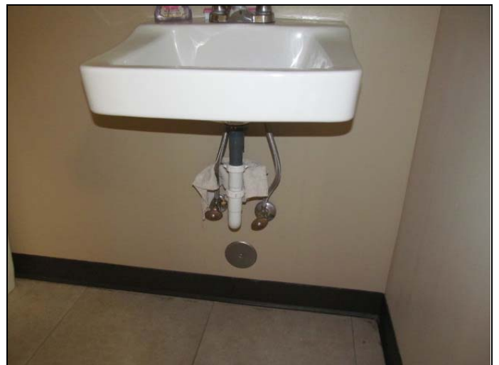
58. Select tenant spaces lacked appropriate scald protection per ADAAG.
