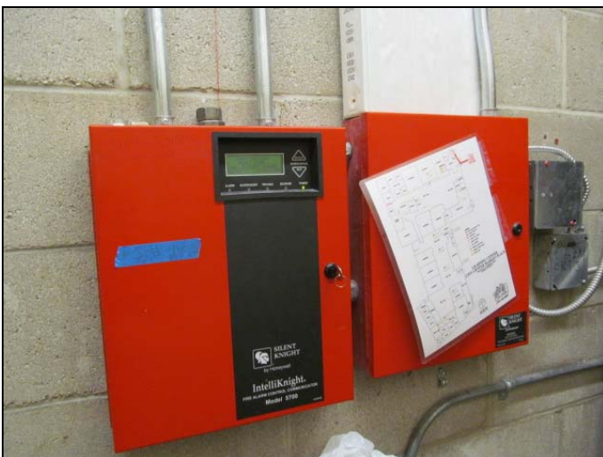
53. View of typical fire alarm control panel.
