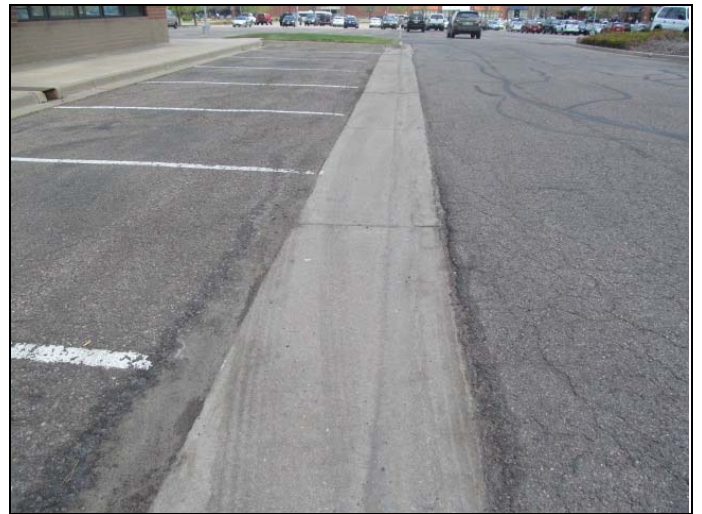
4. View of typical concrete improved drainage swale.
