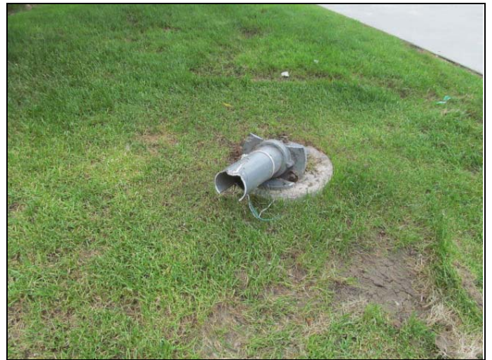
22. View of damaged light pole.
