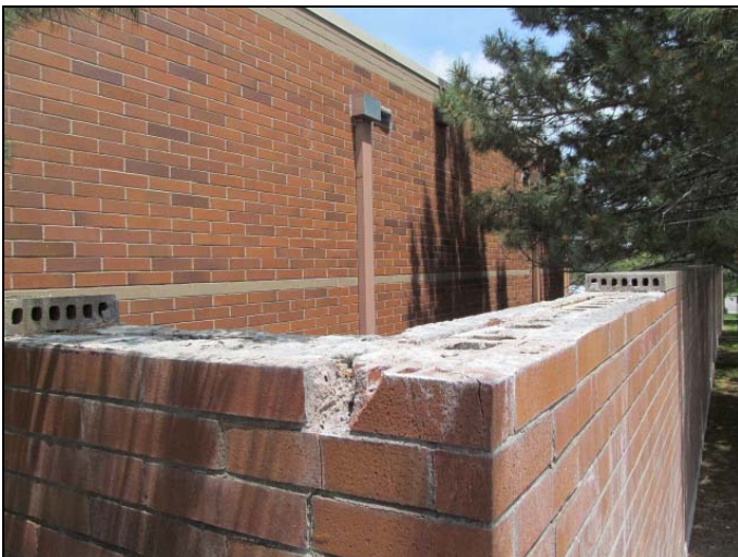
17. View of damaged brick masonry at the wall located at the rear of the 24 Hour Fitness tenant space.
