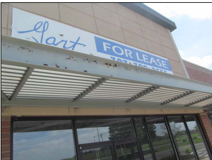
35. View of minor rusting observed at select steel and corrugated metal awning structures.
