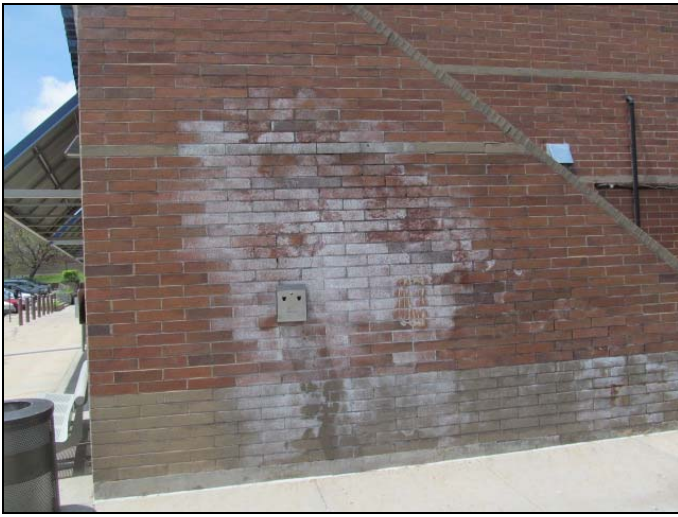
43. View of efflorescence at the exterior stair structure observed at the rear of the 406 South Chambers Road building.
