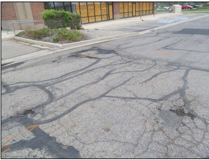
7. View of typical damage observed at the asphalt pavement.
