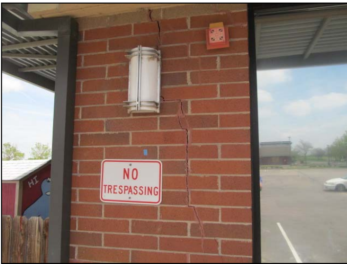
31. View of minor cracking observed at the brick masonry near the entrance to the First Step Infant Daycare tenant space.
