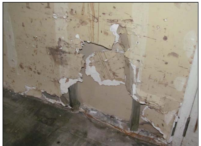
60. View of typical drywall damage observed at vacant tenant spaces.
