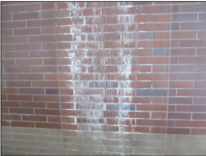
27. View of efflorescence observed at the interior of the exterior brick masonry walls.
