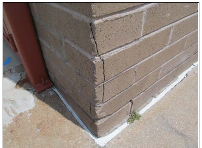
24. View of typical cracking observed at typical trash enclosures.
