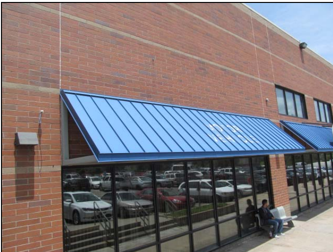
33. View of typical awning structure above tenant space entries.
