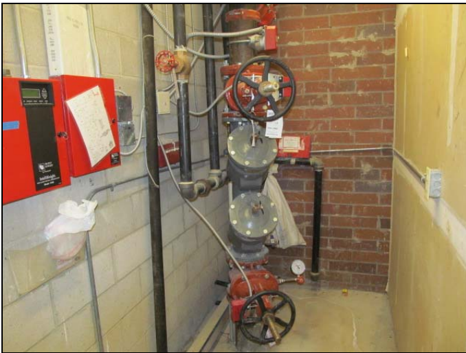
51. View of typical fire suppression riser.
