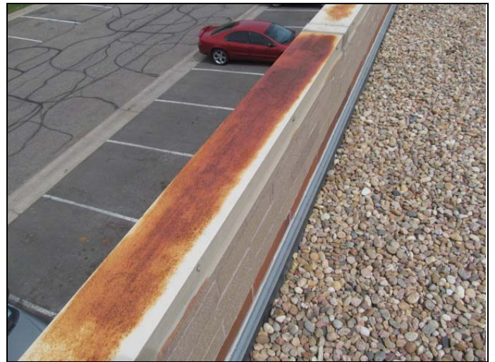
40. View of typical rusting observed at parapet coping.
