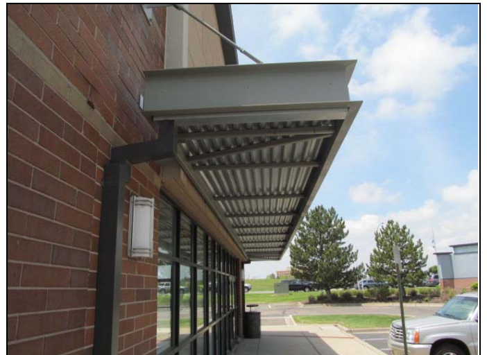
34. View of typical steel and corrugated metal awning structure above tenant space entries.
